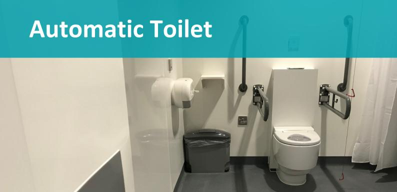
Automatic toilets are not required, but we always recommend them for extra independence. Automatic toilets feature automatic flushing, warm water washing bidet, and warm air dryer.
