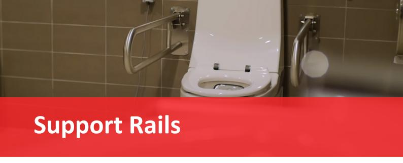
Both wall-mounted vertical grab rails and drop-down support rails should be fixed to the wall either side of the peninsular toilet, to offer support to people while transferring and while seated.
